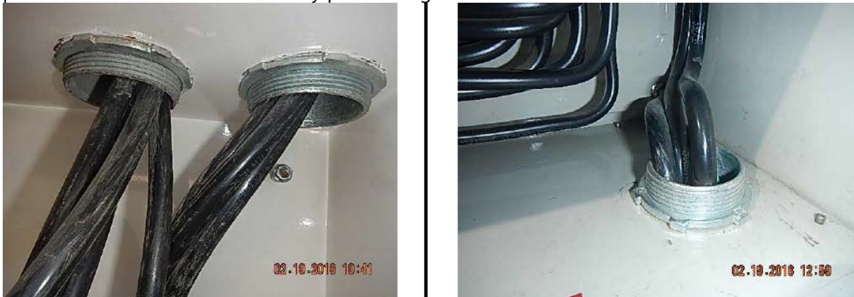
Figure 7: Unprotected raceways in NOX.
