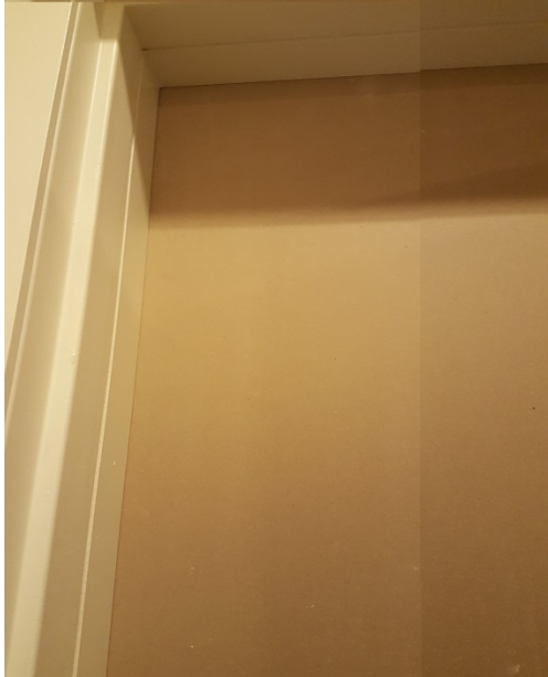
Figure 17: Door connecting two suites in SDA-1 not labeled as having a fire-rated frame.
