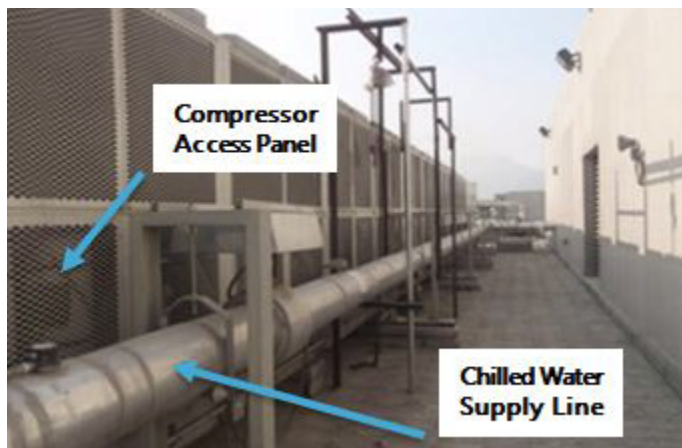
Figure 10: Chilled water line on NOX rooftop.
