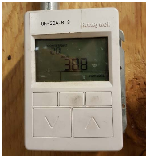
Figure 13: Thermostat in SDA-1 boiler room displaying temperature of 38.8° Celsius (101.8° Fahrenheit). Source: Photo taken by OIG on May 2, 2017.
