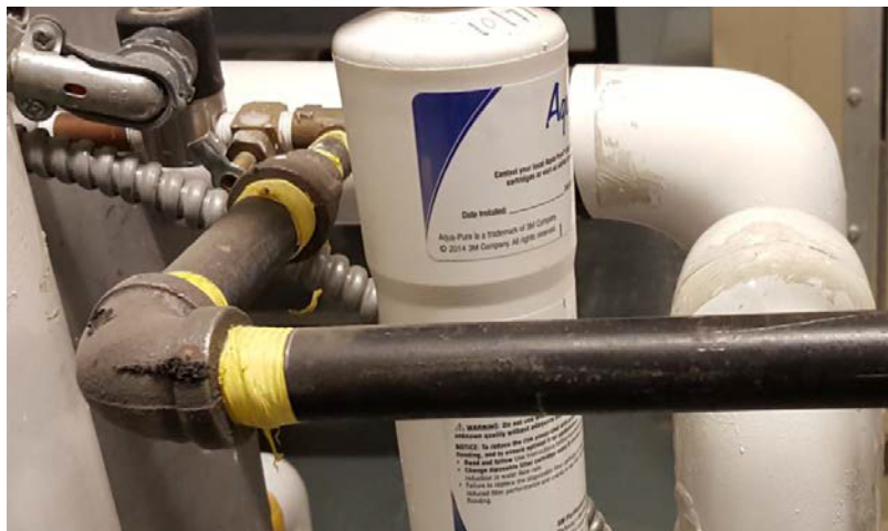
Figure 12: Piping used in HVAC systems in SDA-1 installed without dielectric fittings.
