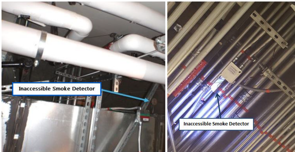
Figure 15: Smoke Detectors in NOX inaccessible for testing and maintenance.
