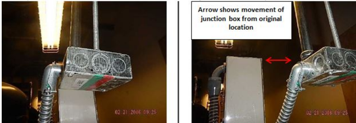
Figure 5: Junction box suspended from the ceiling is not secured properly.
