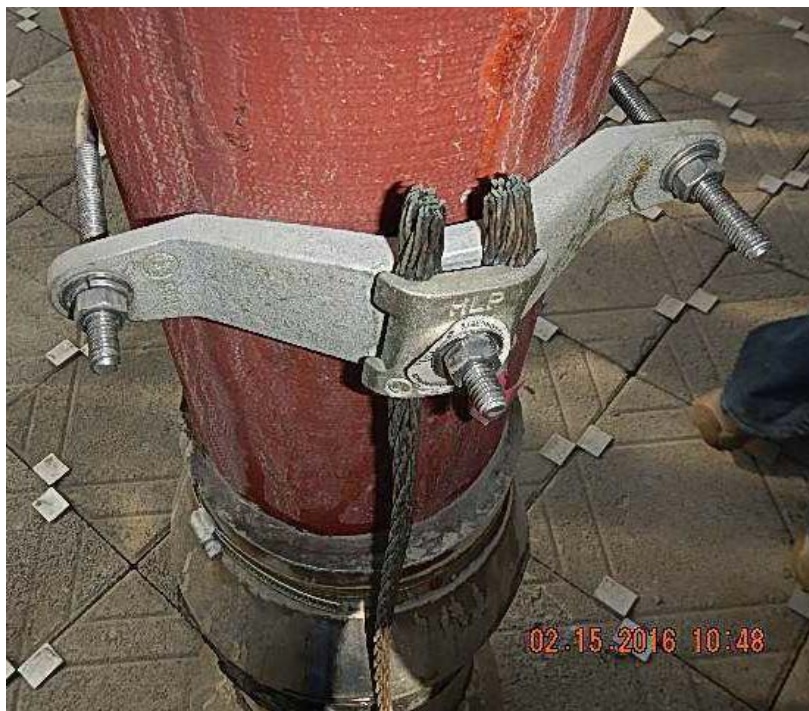
Figure 9: Paint compromises electrical connection with bonding clamp.
