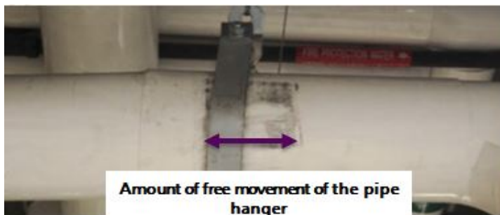
Figure 14: Improper pipe hanger installation.
