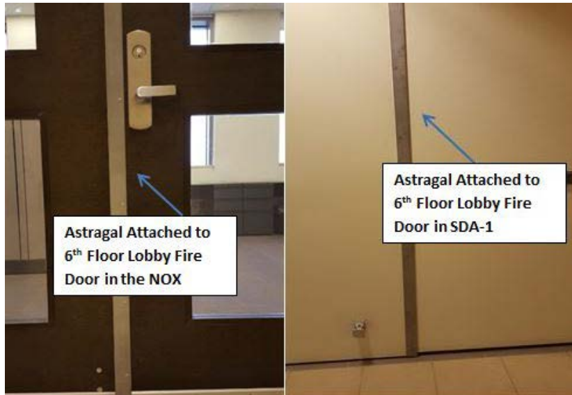
Figure 16: SDA-1 and NOX fire-safety doors with astragal modifications. Source: Photos taken by OIG December 28, 2016, and January 3, 2017.
