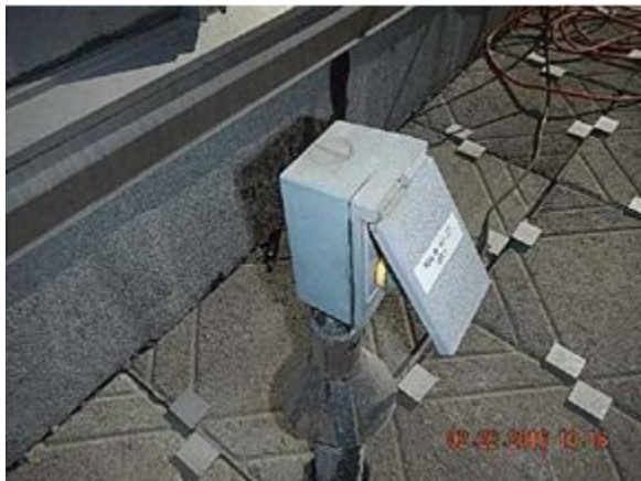
Figure 6: Unattended, plugged-in device without a waterproof enclosure in SDA-1.
