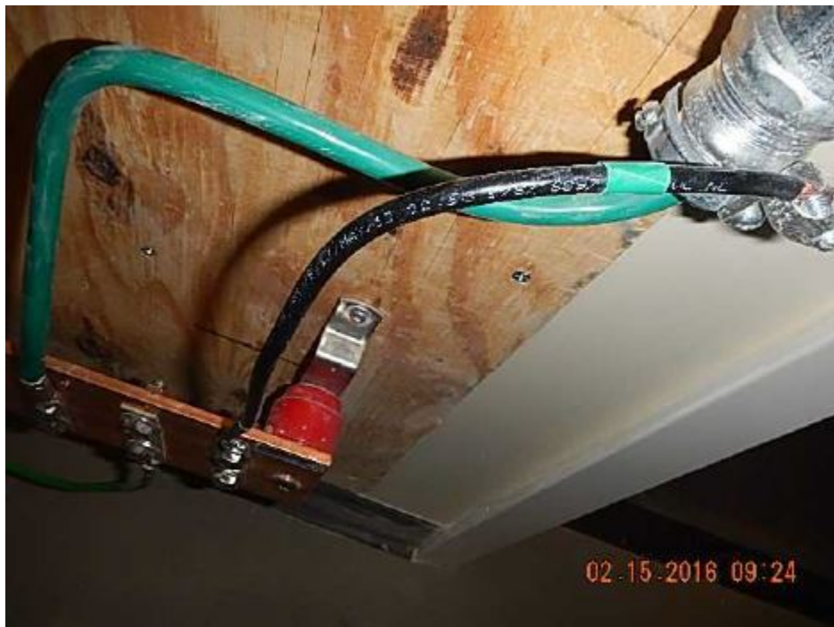
Figure 4: Improper black conductor in NOX labeled with small piece of green tape.
