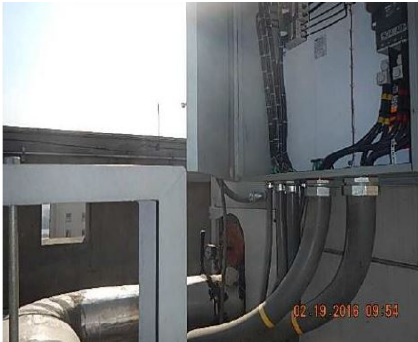
Figure 8: Obstructed electrical panel on NOX rooftop.
