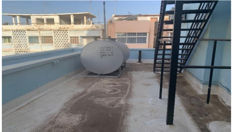
(U) Figure 2: Uncontained fuel tank. (Source: Embassy Praia)
