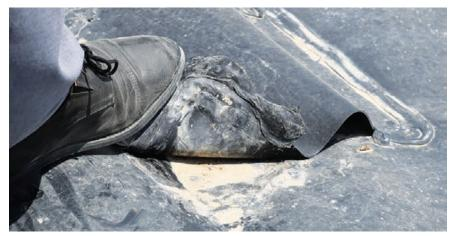
Detached pond liner air vent at wastewater treatment facility. (SIGAR photo)
