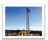
**Integrated Fixed Towers** (IFT) provide long-range, persistent surveillance of rural and remote areas. Each tower is equipped with sensors that continuously detect and track items of interest such as people crossing the border on foot or traveling in vehicles or low-flying aircraft, and provide that information to a Border Patrol command center.
