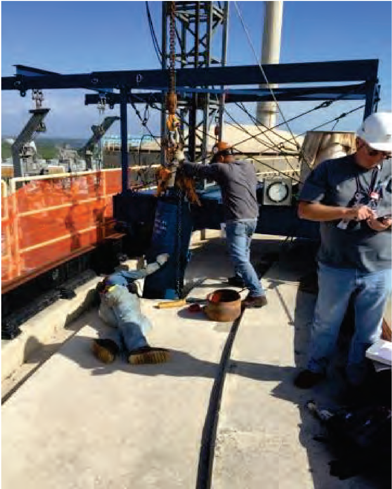
Containment tendon surveillance at the Turkey Point nuclear generating station.
