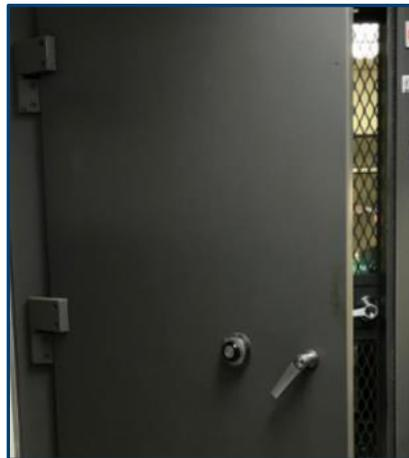
*Figure 1: Pharmacy vault doors, an outer heavy metal and inner cage doors.
