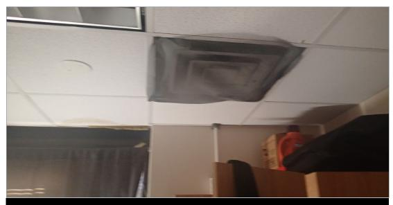
Figure 5. Make-Shift Filter on Dorm Room Air Return in Building 106 Source: The DoD OIG.
