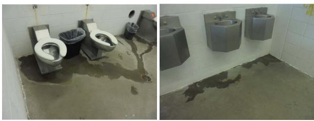
Figure 2. Detainee sinks and toilets leaking water observed by OIG at El Paso on April 30, 2019. *Source:* OIG
