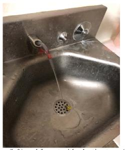
Figure 5. Leaking faucet without plastic straw (left) and faucet with plastic straw (right) observed by OIG at Baker on July 30, 2019.
