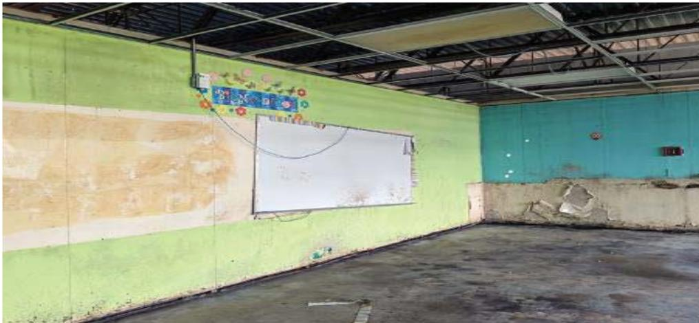
**Figure 1: Classroom with molded floors and water-damaged walls at a school in San Juan, Puerto Rico**
