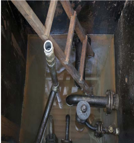
Figure 1: Water on top of the diesel storage tank at Embassy Ankara, Turkey. (OIG photo, Oct. 2018)
