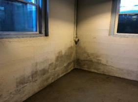
Figure 7. Potential Mold on Basement Wall
