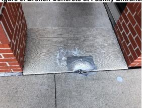
Figure 9. Broken Concrete at Facility Entrance
