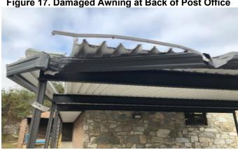
Figure 17. Damaged Awning at Back of Post Office
