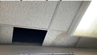
Figure 5. Missing Ceiling Tile
