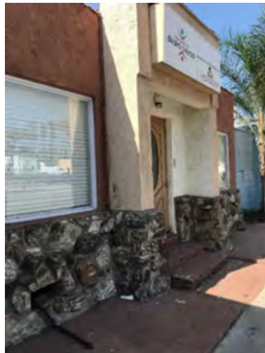
Foundation for Second Chances building
