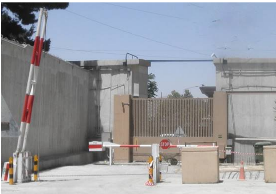
(U) Figure 2: Vehicle gate and reinforced wall at Embassy Kabul. (Photo taken by OIG, July 2018)
