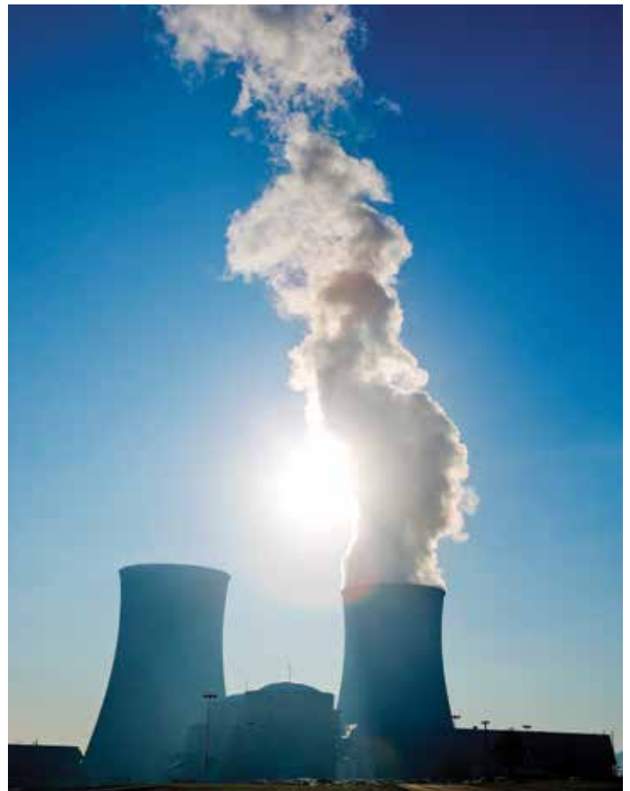
Watts Bar Nuclear Plant
