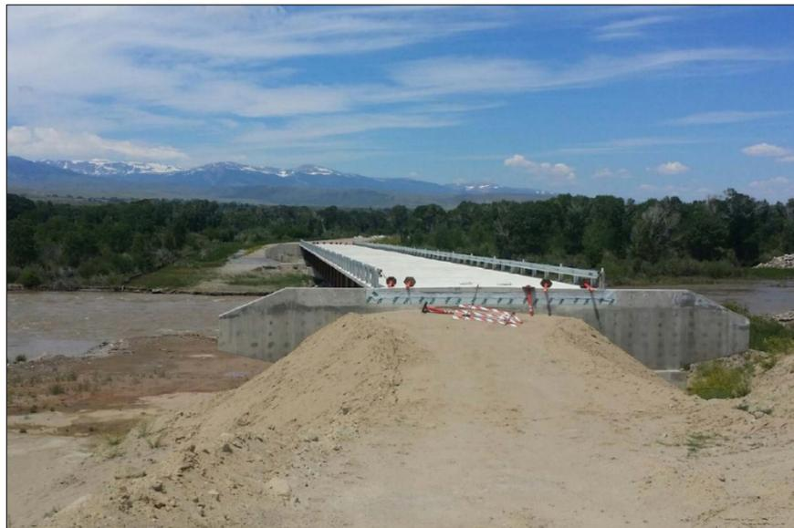
Figure 1. The Lenore Bridge project has not been completed, as the approaches still have not been constructed. Source: OIG.
