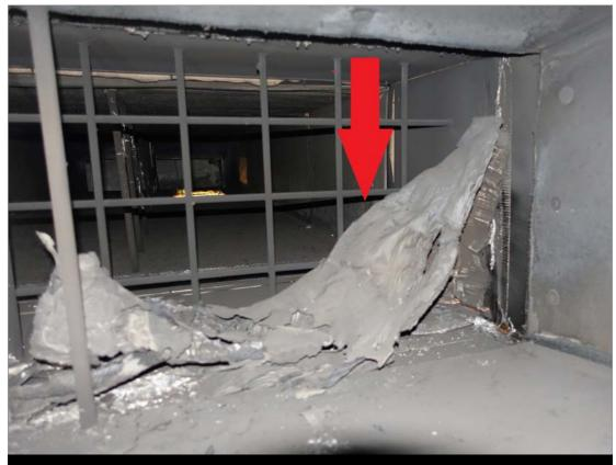
Figure 4. Charred Cardboard Left in the Ductwork Source: USACE Omaha District.
