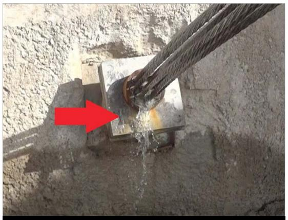
Figure 2. Water Leaking from the PERS Wall Source: USACE Omaha District.
