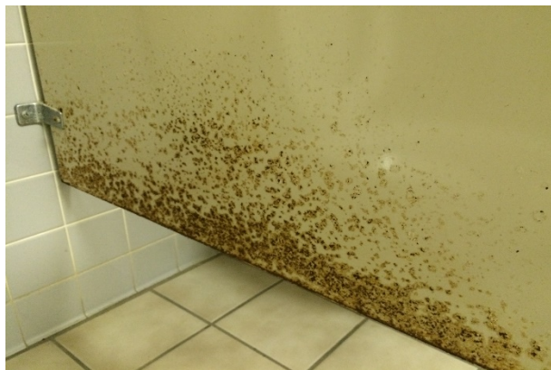
Photograph 1: Peeling paint revealing rust covering a bathroom stall divider.
