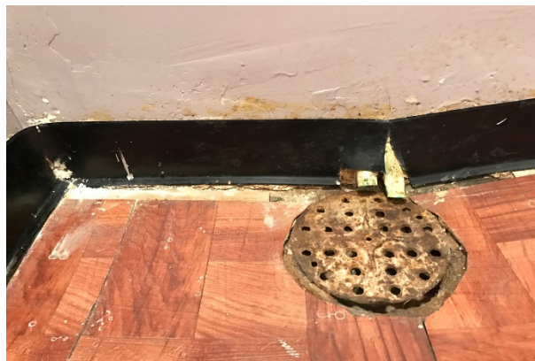
Photograph 2: A rust-covered floor drain and peeling paint in a bathroom.
