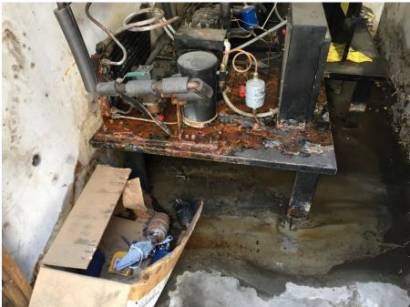
Images 4, 5, and 6: Mold spores and water-damaged refrigeration equipment - Spearly Care Center
