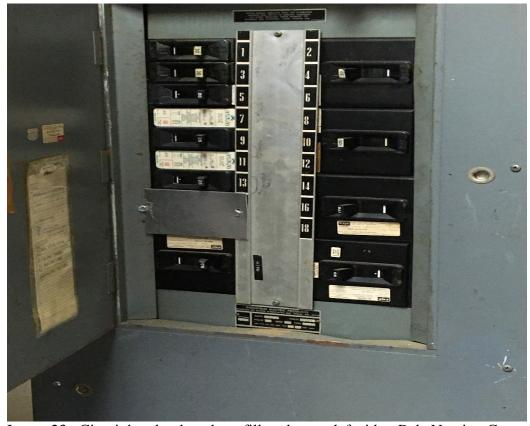
Image 23: Circuit breaker knockout filler plate on left side - Bala Nursing Center
