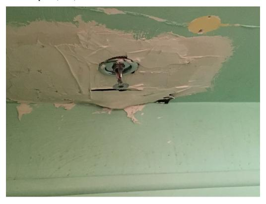
Image 22: Repair not compatible with design and quality of the original and joining decorative materials - Spearly Care Center
