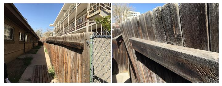
Images 2 and 3: Fencing leaning and sections damaged - Spearly Care Center
