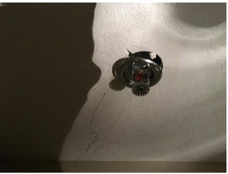
Image 9: Damaged fire sprinkler escutcheon - Cherry Springs Village
