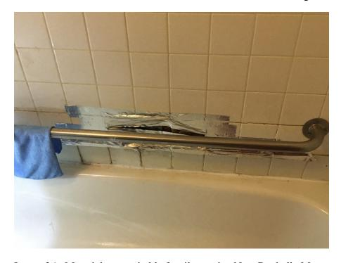
Image 26: Materials not suitable for tile repair - New Rochelle Manor
