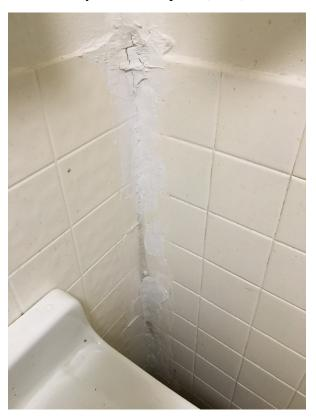
Image 24: Repair not compatible with design and quality of the original and joining decorative materials - New Rochelle
