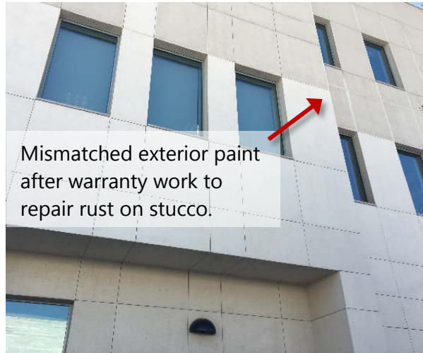
Figure 4: Mismatched paint on exterior wall of support annex. Photo taken February 13, 2017.
