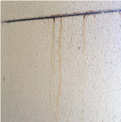
Figure 3: Rust bleeding through stucco and running down exterior wall of Marine security guard quarters. Photo taken February 13, 2017.
