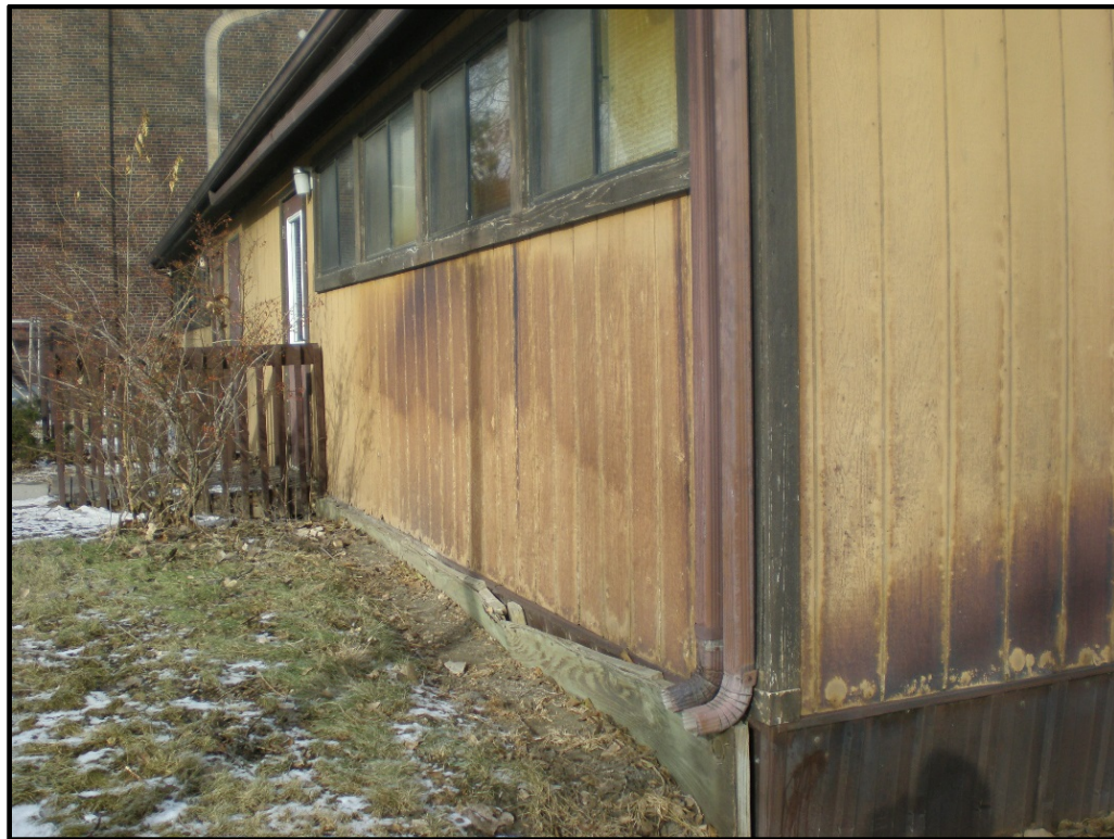
Figure 12. Pierre Indian Learning Center portable in visibly poor condition, with damaged walls, gutters, roof, and window treatments.
