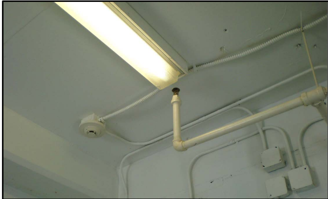
Figure 13. A sprinkler head at one school that was installed so it aims directly at an adjacent lighting fixture.
