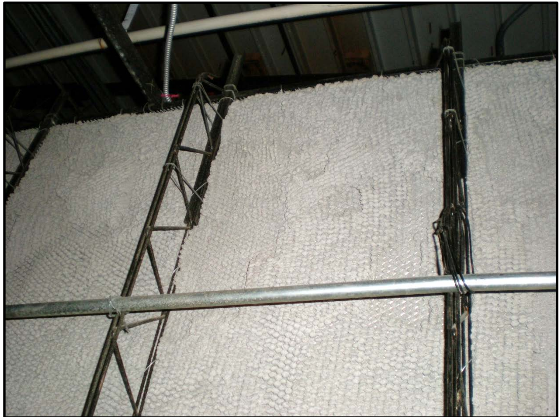
Figure 7. Thick walls of asbestos insulation are left in one dormitory because the cost to remove it is "outrageous."
