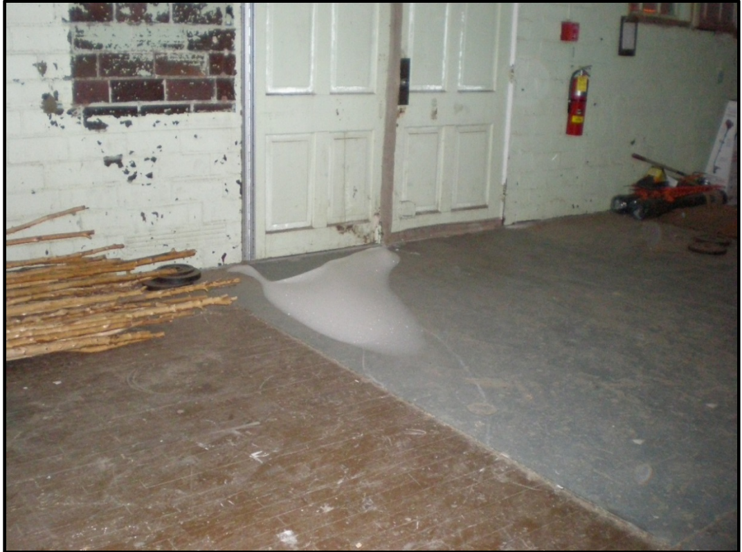
Figure 9. Building space is needed for student activities at Flandreau Indian School so this building is kept from being demolished even though parts of the building have been torn out and the doors allow snow to enter.
