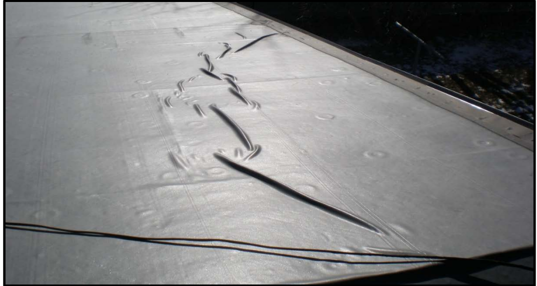
Figure 5. Rolls in the new roof at Rosebud Dormitory indicate poor quality installation and increase the likelihood of future problems.
