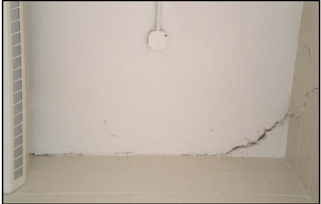
Figure 8. Structural cracks in the stairwell ceiling at Flandreau Indian School.
