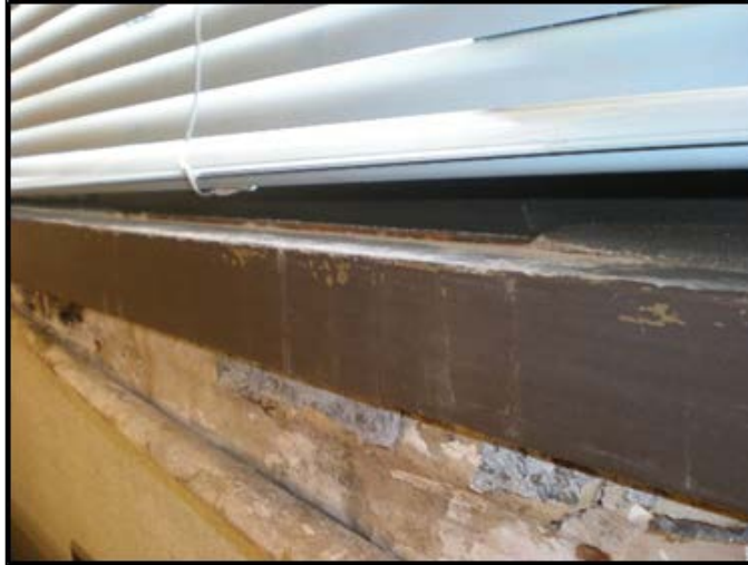
Figure 5. Water damage and mold around a window in the library. Source: OIG
