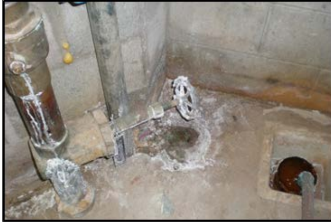
Figure 6. Corroded pipes in the gymnasium. Source: OIG
