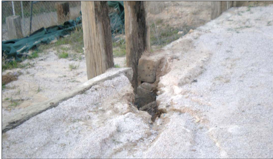
Figure 11. A retaining wall installed in the new building is already structurally compromised. Source: OIG
