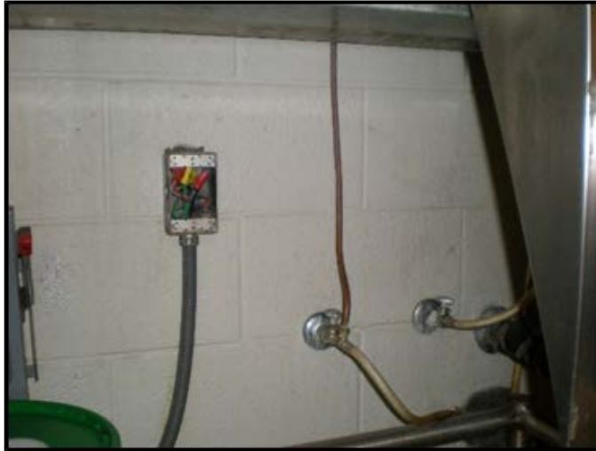
Figure 2. Improperly protected wires under cleaning equipment and near water lines in the kitchen in the cafeteria. Source: OIG
