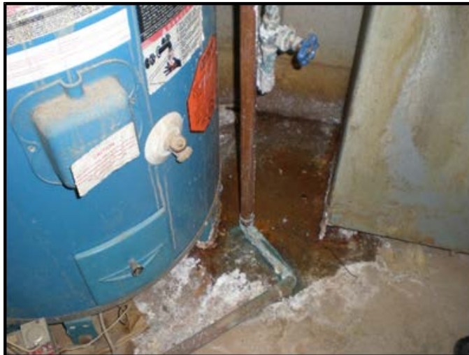
Figure 4. A water heater in the gymnasium was leaking. Source: OIG
