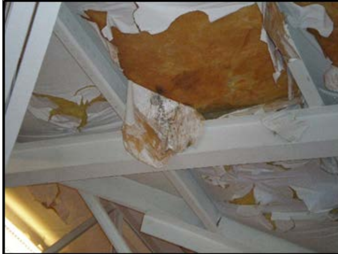
Figure 3. Water damage and mold indicated in the ceiling of the gymnasium. Source: OIG
