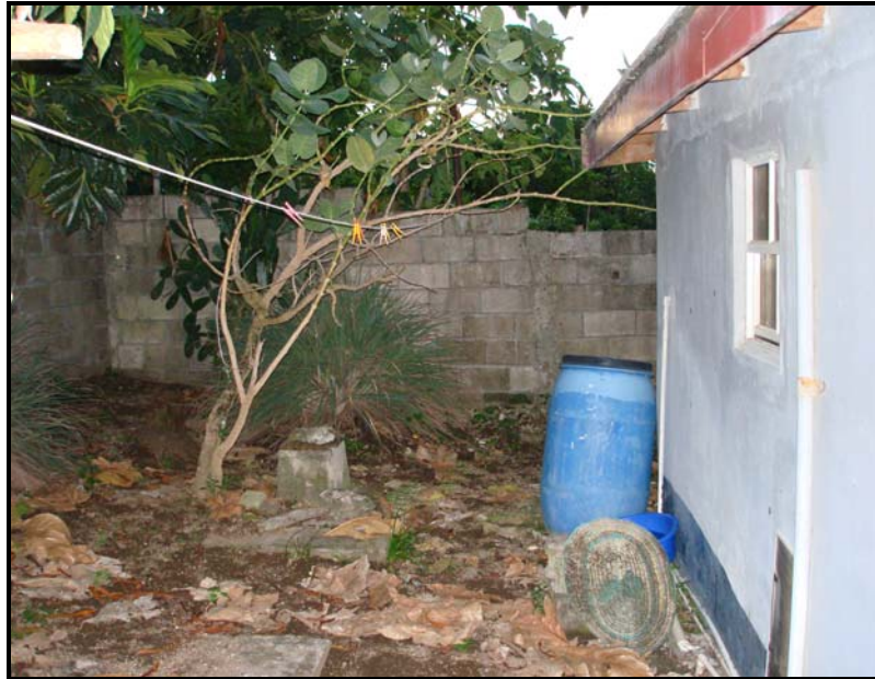
Figure 5. Volunteer's House on St. Kitts
