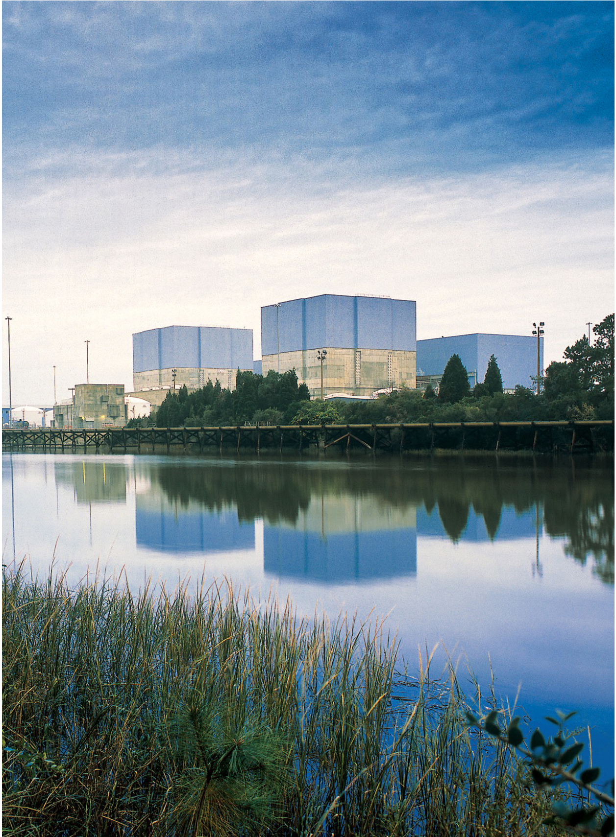
Brunswick Nuclear Power Station. Photo courtesy of Progress Energy
