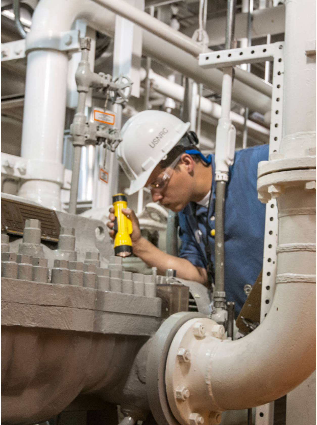
Resident Inspector performs a walk through inspection at Calvert Cliffs nuclear power station.
