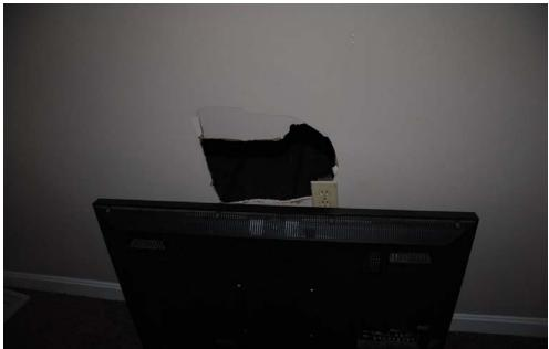
The picture above shows a large hole in the drywall of a bedroom.
