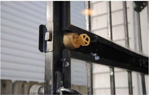
The picture above shows a keyed deadbolt lock on the unit's rear security door. The exit would be blocked in case of emergency if the tenant could not find the key.
