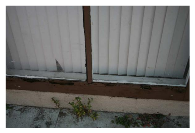
The picture above shows a unit with window conditions involving a deteriorated, damaged, and rotting window frame and an improper weather-tight seal. In addition, the window did not have
