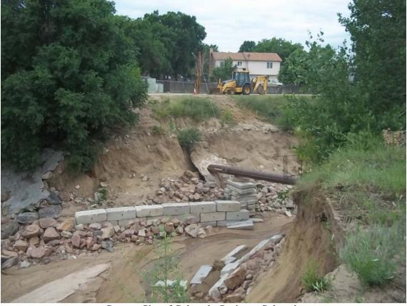
Figure 1: East Fork Sand Creek Channel Failure
