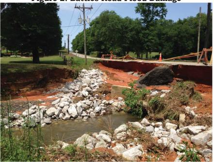
Figure 2: Battles Road Flood Damage
