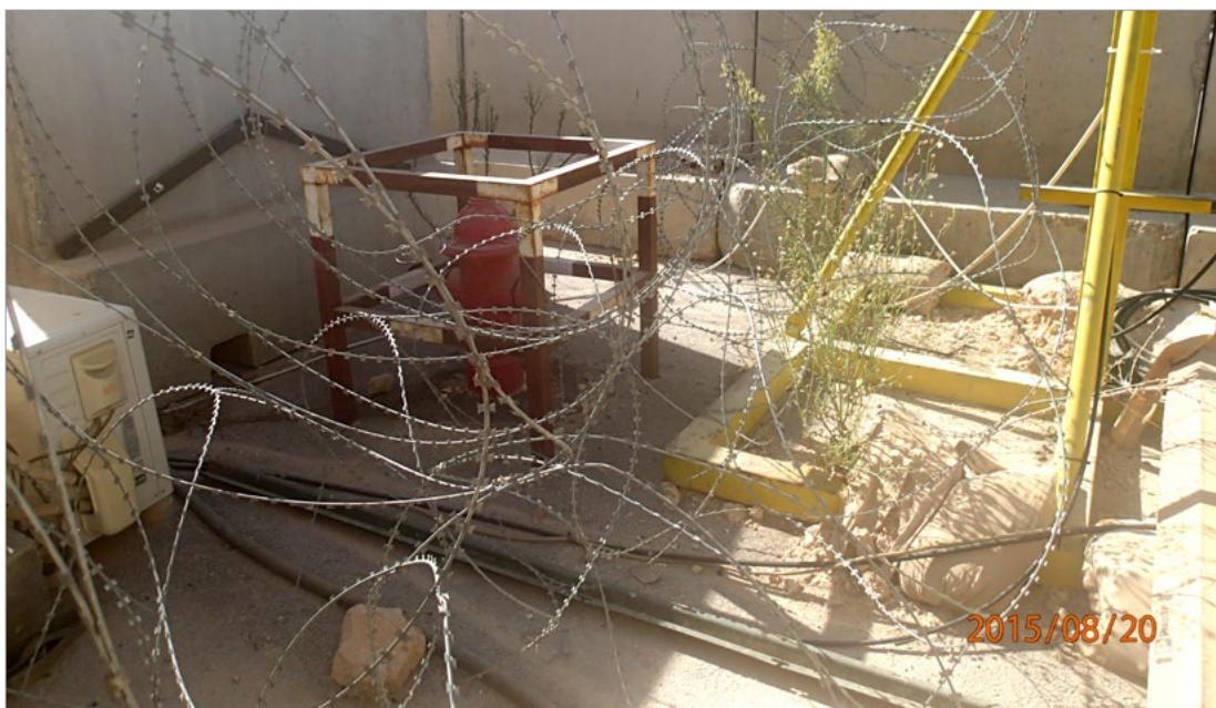
Figure 7. Obstructed fire hydrant at KASOTC, Jordan. (Deficiency No. KAS-FP-150828-137) Source: Report No. DODIG-2016-106
