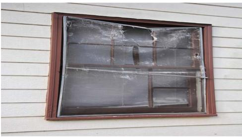
This picture shows a bent frame and torn screen on a window. The tenant could not open the window without letting insects and debris into the house.
