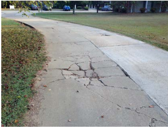
Pot holes in the parking lot.
